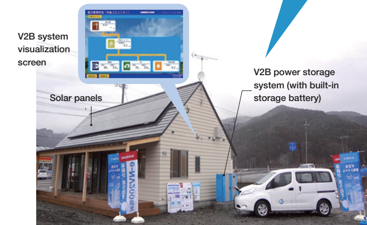
Otsuchi Community Place and V2B power storage system
