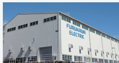
New raw strip plant
