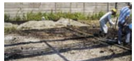
Chiba Works / Work of replacing soil
