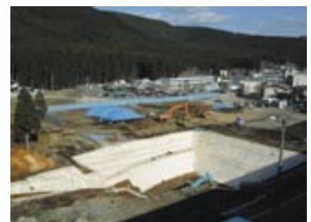
Site of countermeasures taken for contaminated soil at Tochigi Metal
