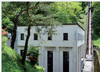
Uwanoshiro Power Plant
