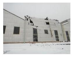
Collapsed roofing immediately after the snow damage
