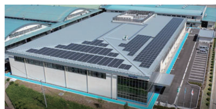
Solar power panels installed by TOTOKU Electric Co., Ltd. (started operation in January 2021)
