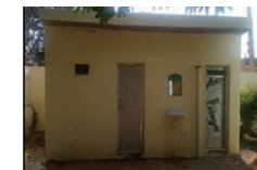
Providing sanitary facilities to schools (Furukawa Minda Electric Private LTD. )
