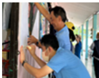
Repainting the walls of a local elementary school in 2023 (FAST*)
