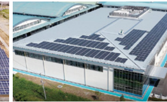
Solar power generation panels installed by Totoku Electric Co. (operation start, January 2021)
