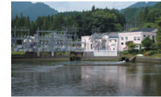
Furukawa Nikko Power Generation hydroelectric power generation
