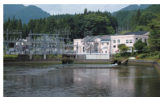
Furukawa Nikko Power Generation hydroelectric power generation
