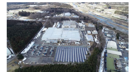
Solar power generation panels installed at the Imaichi East Plant of the Copper Foil Division (operation start, February 2019), and introduction of electricity derived from renewable energy (operation start, April 2022)
