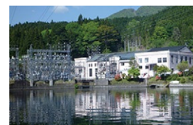
Furukawa Nikko Power Generation Inc.’s hydroelectric power generation
