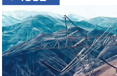
Completed large-scale power transmission line installation in Iran
