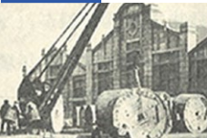
Started manufacturing electric copper wires
