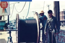
Installed a communications network in Bangkok, Thailand
