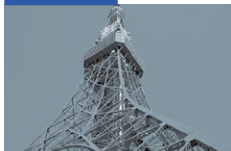
Installed an antenna and feed line on Tokyo Tower
