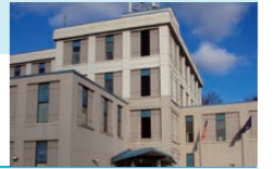
Acquired SuperPower Inc., a high-temperature superconducting materials manufacturer in the US
