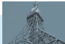
Installed an antenna and feed line on Tokyo Tower
