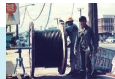
Installed a communications network in Bangkok, Thailand
