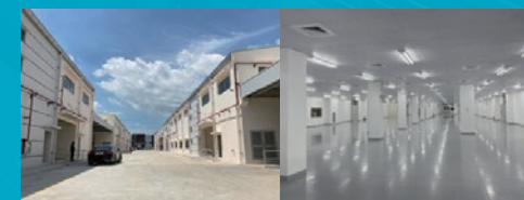
Manufacturing plant for data-center water-cooling modules FURUKAWA ELECTRIC THERMAL MANAGEMENT SOLUTIONS & PRODUCTS LAGUNA, INC. (Philippines)
